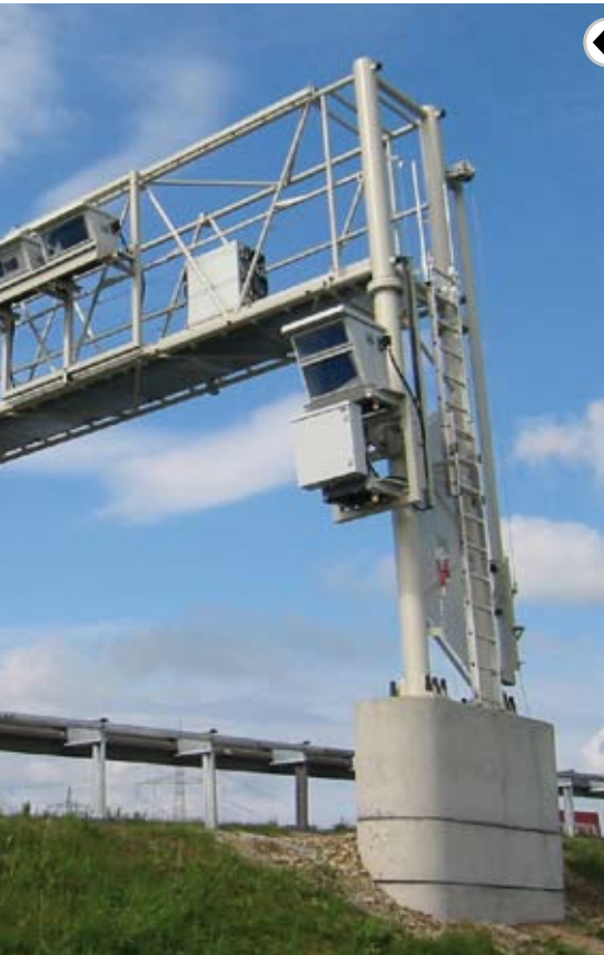
Vitronic's TollChecker is a major part of the German truck-tolling scheme, enforcing the correct payment of tolls
